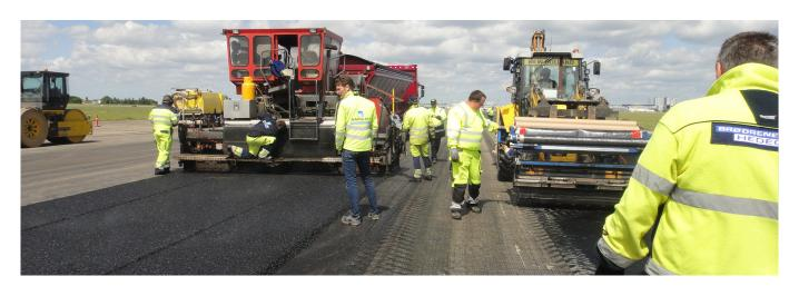
▲ Mechanical unrolling of S&P Carbophalt <sup>®</sup> G in one of the busiest areas of the airport and application of new asphalt pavement onto the S&P grid
